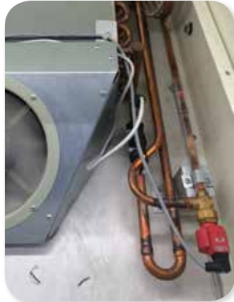
Electronic expansion valve for the evaporator
